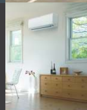
Air conditioning: Split A/c for all the bedrooms.
